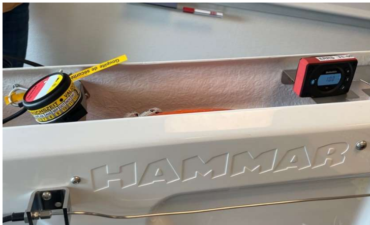
Detailed view of a ERU electronic unit at 10° inclination inwards
